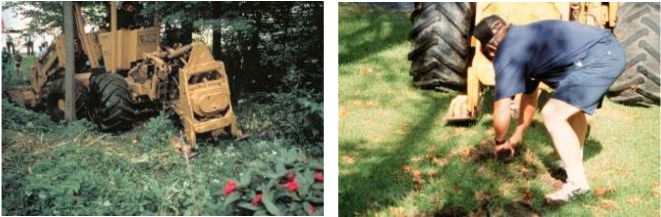
Figure 5. A. Vibratory plow operating in tight conditions. B. Sod being repositioned after tree roots were disrupted by a Vibratory plow.
