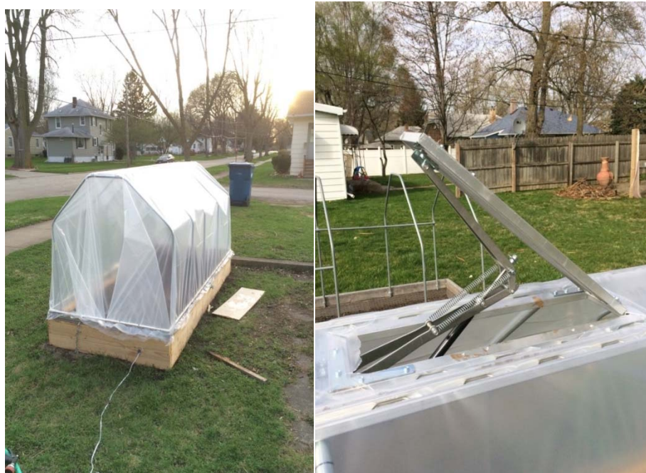
Left: ½" EMT hoops bent at two 45-degree angles to form a 4-foot wide hoop. These serve as the basic structure. Right: Automated vent arm to control temperature and humidity in mini-tunnel.
