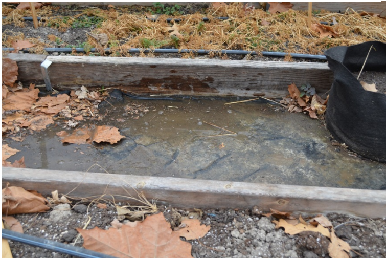
Ahoy! The high tunnel has a couple inches of standing water from two days of winter thunderstorms. Photo: C. Enroth.
