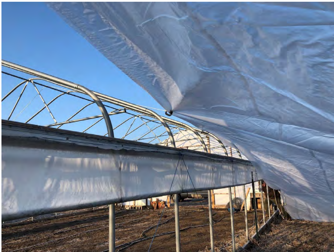
Pulling the new top on the high tunnel. Photo by Dusty Spurgeon
