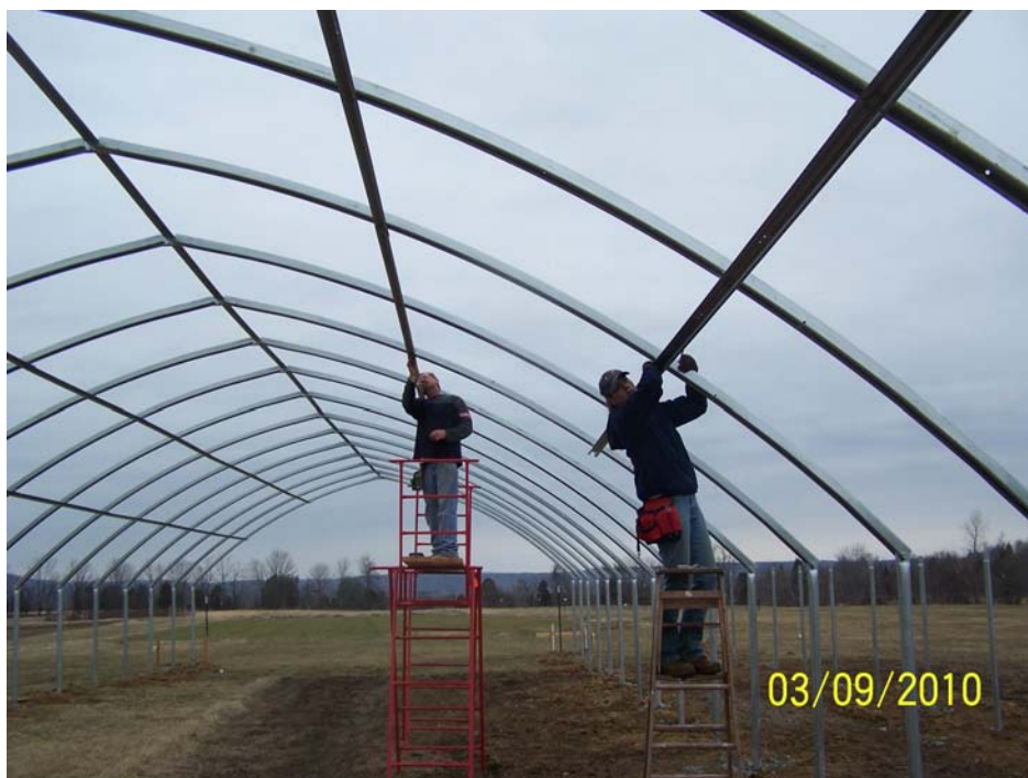
One of the new high tunnels under construction at DSAC.
