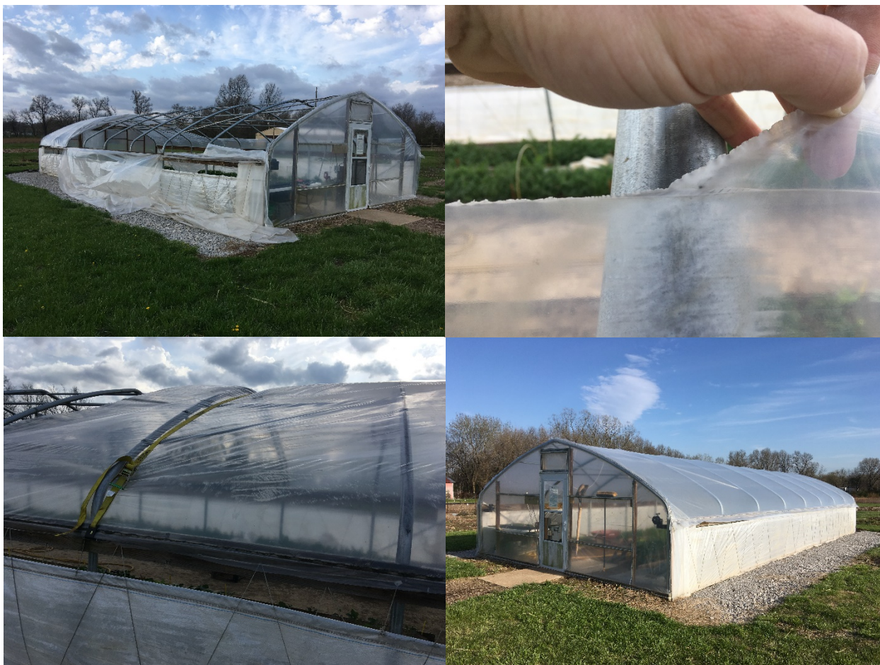
Plastic torn off by the wind on the research high tunnel at the Jackson Co. office. (top left). 4 and a half year old plastic failed right along a crease from the manufacturer. (top right). Using a ratchet strap to stabilize remaining plastic until the weather allowed to make further repairs (bottom left). New plastic on, trimmed and we are back in business! Photos: N. Johanning.
